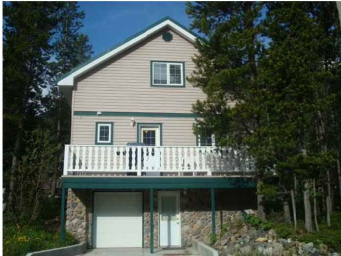
Back Elevation (Looking from Parking Lot)
