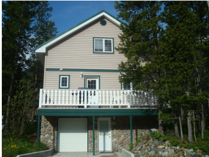
Back Elevation (Looking from Parking Lot)
